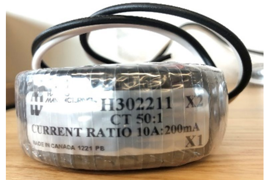
Fig. 7: Current transformer made by Hammond Manufacturing.
